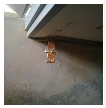
Vandals started to steal the earth cables from primary sub-stations which is consider as high danger. Such thefts will cause complete damage, fires and expulsion of transformers and other assets like switchgear and protective relays.
