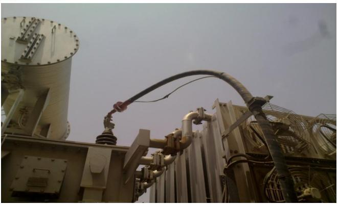
For the purpose of stealing the bus-bar and neutral cable vandals connect the neutral cable with the earth cable. By that act personal and asset will be in major danger of transformer fire and explosion
