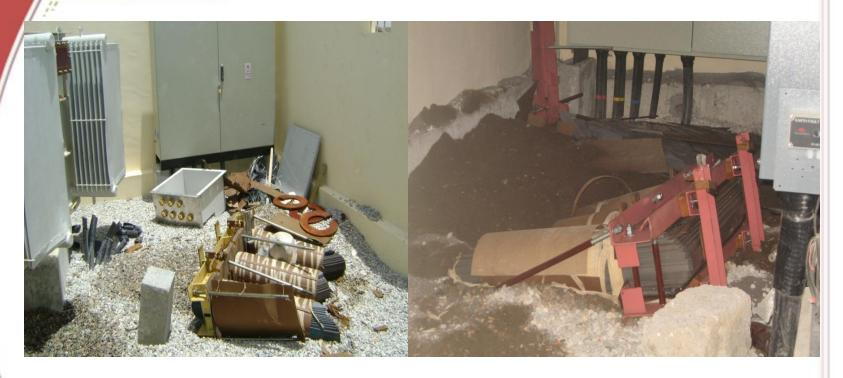
These transformers contain windings which are made of pure copper and consider as the most target for theft due to the high price of stolen copper
