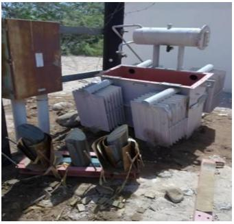
The main target in such transformer is the winding which also made of pure copper. Vandal's shutdown the transformer by pulling the Dropout Fuse (DO FUSE) After that, they drop the transformer to the ground and steeling the copper.
