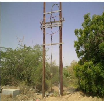
In such theft vandals pull the Dropout Fuse (DO Fuse) to isolate the line then they took the copper from the cable (3 core 240 mmsq).
